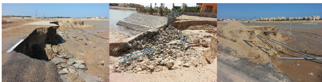
Figure 1. Collapse of infrastructure due to the scour effect: main road (left), bank protection (middle), and cutting lines of electricity, internet and phone (right) (Helal, 2014)
